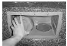
Install Eco Pur filter on left side.
